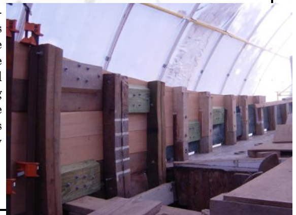
The newly cut sheer lines show some real progress
